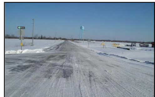
Low Volume Road Plowed for Two-Way Traffic
