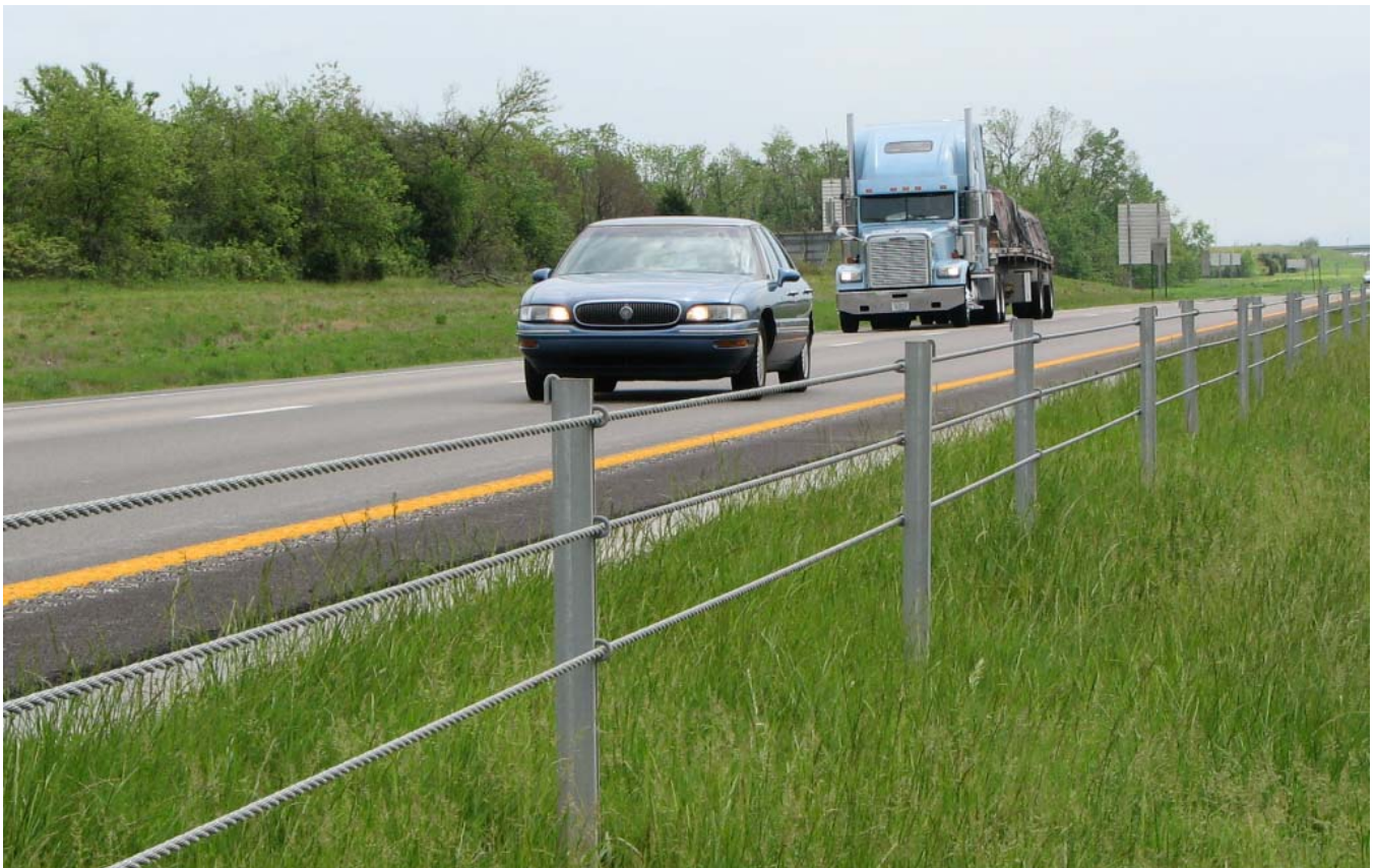
FIGURE 2 High-tension cable median barrier
