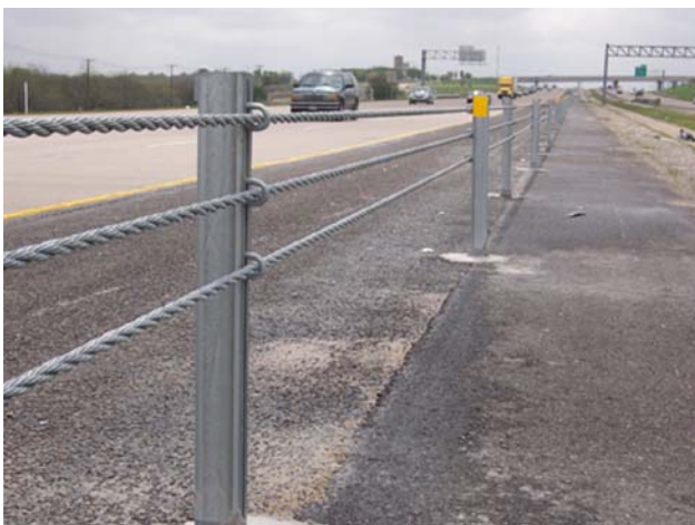
FIGURE 4 Asphalt vegetation control apron
