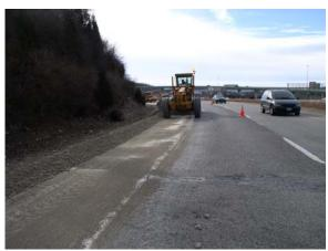
(15) Blading 2" Aggregate with Motograder
