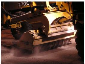
(1) Roto Grader Milling a Pavement Joint
