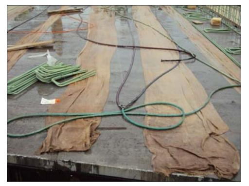
Figure 11 - Good Grout Curing
