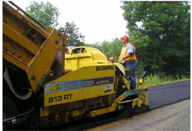
(2) Self Propelled Paver
