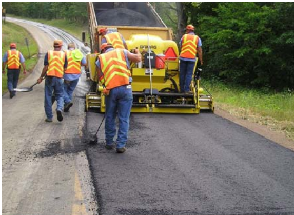
(3) Hand Raking as needed
