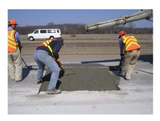
(10) Machine Finish Concrete with Bunion Tube
