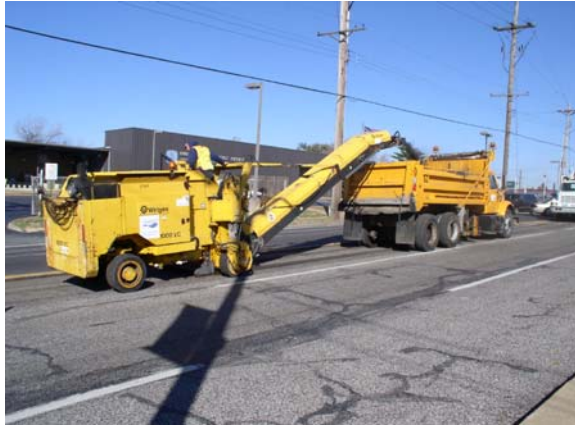
(1) Pavt Repair Milling Operation
