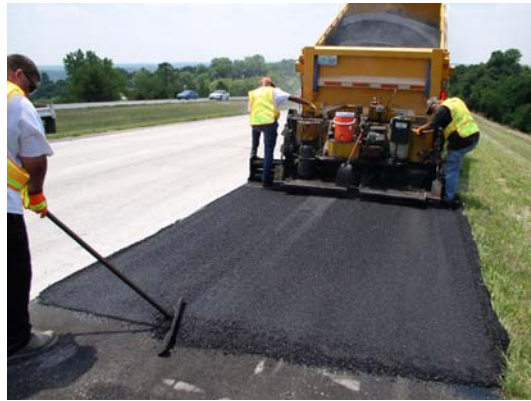
(2) Box Spreading Hot Mix Asphalt
