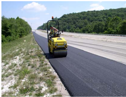
(4) Rolling Hot Mix Asphaltic Shoulder -- Finished Product
