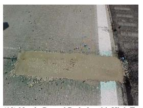
(10) Newly Poured Pothole with High Type Patching Material
