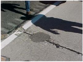
(7) Deteriorated Concrete Joint/Spall
