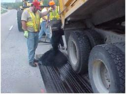
(4) Laying Asphalt on prepped area
