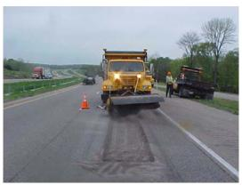
(3) Sweeping a section of partial depth milled asphalt
