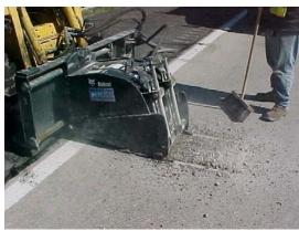
(8) Preping Pothole with Milling Attachment
