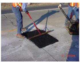
(16) Raking Hot-Mix into Pothole
