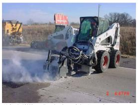
(12) Milling Pothole with Attachment
