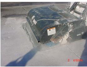
(14) Sweeping Concrete Pavement Pothole
