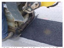
(5) Finishing Partial Depth Asphalt Patch (6) Finished Product
