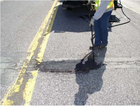
(15) Sealing Pothole Patch
