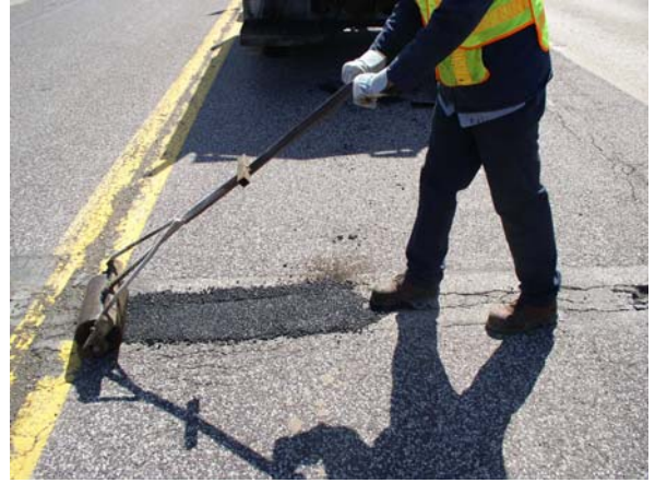
(14) Hand Rolling Pothole Patch
