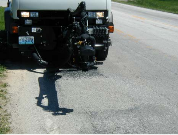
(7) Injection Patcher Set Up
