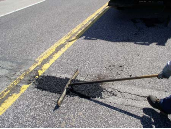
(13) Leveling Pothole Patch
