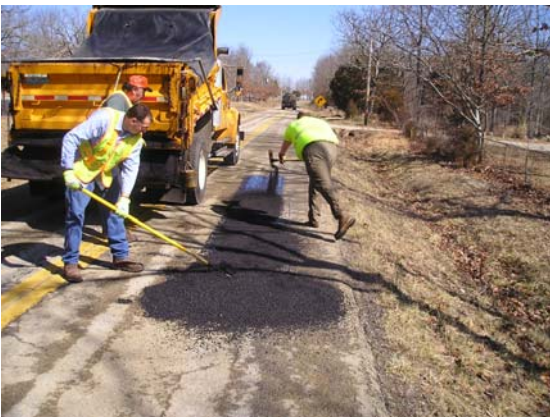
(5) Applying Cold Patch
