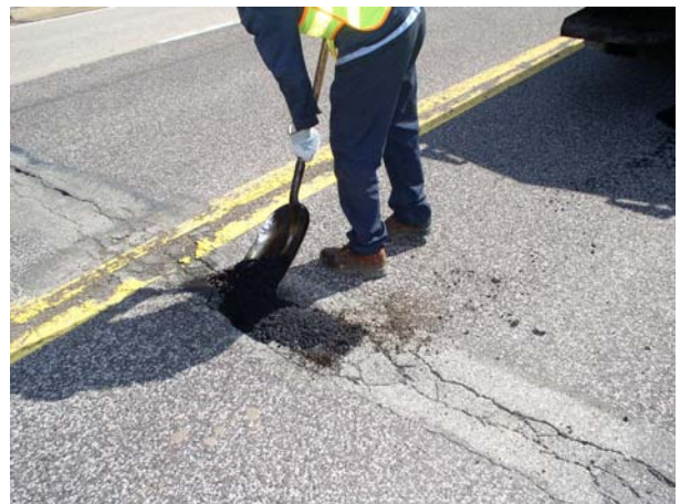
(12) Filling Pothole with Cold Mix Asphalt
