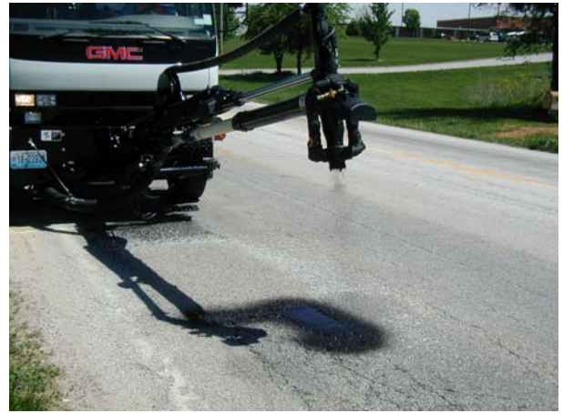
(8) Injection Patcher Application
