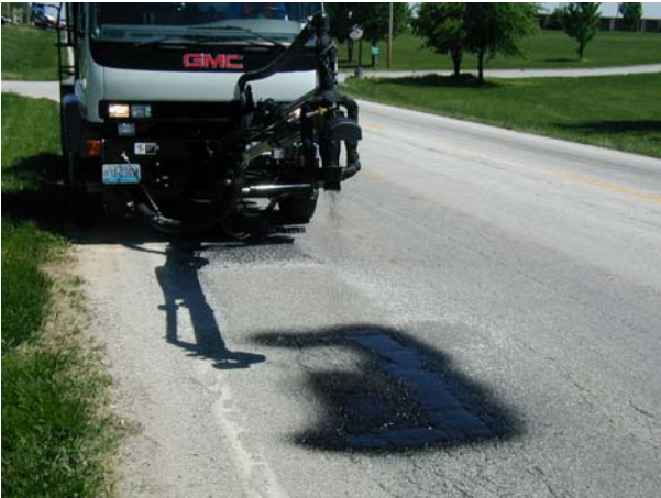
(9) Injection Patcher Application
