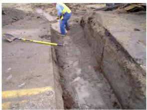
(4) Fine Grading Culvert Bed
