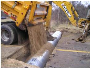
(7) Backfilling around Culvert Pipe
