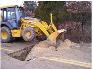
(8) Spreading and Compacting Pipe Fill
