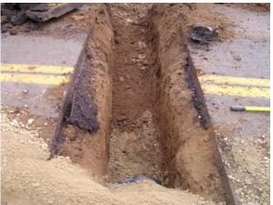
(2) Open Trench for Culvert Replacement
