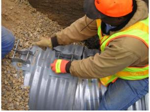
(6) Installing Pipe Connecting Band
