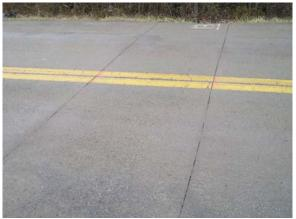
(1) Sawcut Pavement for Culvert Replacement
