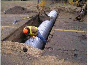
(5) Laying Culvert Pipe
