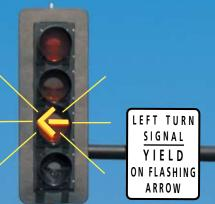
The Missouri Department of Transportation is implementing a new traffic signal display to provide a safer, more efficient left turn for motorists. The flashing yellow arrow left-turn indication is a new type of display that can replace the circular green indication for left turns at selected signalized intersections.
