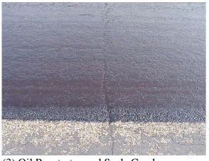
(3) Oil Penetrates and Seals Cracks
