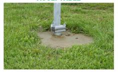
Concrete is flush with surrounding finished grade and the breakaway ground anchor set in the concrete is less than 4" above the finished grade and concrete.
