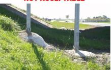
Concrete is poured above the level of the surrounding ground elevating the fixed portion of the breakaway device above the maximum 4" above the surrounding finished grade
