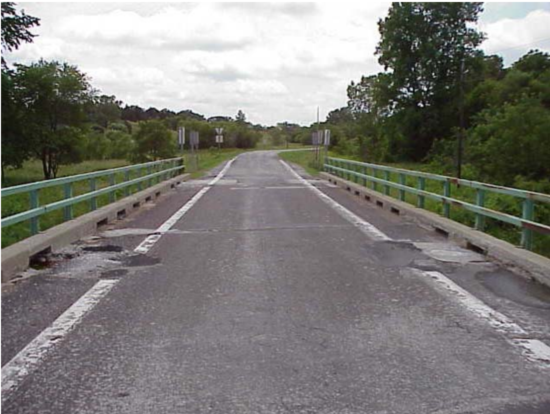
View of bridge before replacement.
