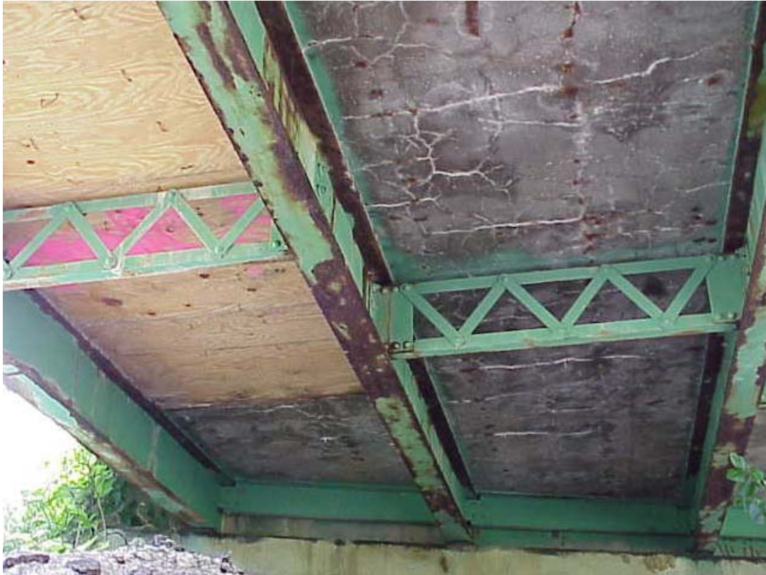
View of girders and underneath side of deck.
