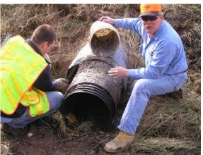
(10) Grouting Pipe Liner to Culvert End
