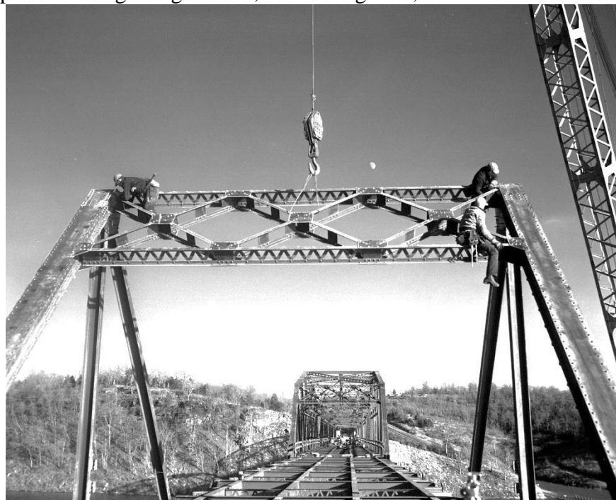
Figure 1: Portal bracing being erected, Theodosia Bridge, Ozark County
