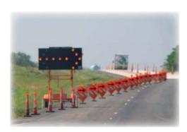
Temporary traffic control devices are the medium through which traffic is informed of and guided through a temporary traffic control zone or otherwise protected from an unsafe condition. The most common devices include signs, portable changeable message signs, flashing arrow panels, channelizers, barricades, temporary traffic barriers, pavement markings, lighting devices, temporary traffic signals, crash cushions, protective vehicles and truck-mounted attenuators.
