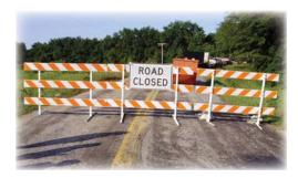
A barricade is a portable device used to close, restrict or delineate all or a portion of the right of way to motorized and non-motorized traffic. Each unit contains a number of rails augmented with stripes of alternating orange and white retroreflective sheeting on the side facing traffic.
