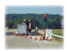
Temporary traffic control signals are used at haul road or equipment crossings, on one-lane, two-way operations, and at temporary intersections located within the temporary traffic control zone to assign vehicular right of way. Typically, this is done with temporary span-wire installations or trailer-mounted units.
