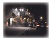
nighttime operations by illuminating the work area to a level at which workers can adequately see what they are doing. A minimum intensity of five footcandles is recommended to satisfy this objective. Typically, this lighting is provided by an array of vehicle- or equipment-mounted floodlights, an array of floodlights on a portable lighting unit, or an internally illuminated balloon. Lighting shall be positioned so that it does not cause glare for motorists, spill onto adjacent properties,
