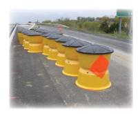
Crash cushions are systems that mitigate the effects of errant vehicles impacting roadside obstacles such as fixed objects or exposed barrier and guardrail ends. The system is designed to accomplish this by either smoothly decelerating the vehicle to a stop or redirecting the vehicle.
