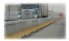
Due to the amount of resources needed to put barrier in place, this option is generally reserved for long-term stationary operations where the need for the noted functions is critical.
