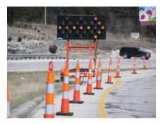
For stationary lane closures, the panel should be deployed on the shoulder or within an adjacent closed lane at the beginning of the lane or one-lane, two-way taper. Where adequate space or the temporary traffic control plan does not permit this placement, the unit may be placed within the taper of the closed lane. When closing multiple lanes, a separate unit shall be used to close each lane.
