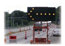
capable of flashing displays. The devices are intended to provide additional warning and directional information to assist in traffic movement through or around a temporary traffic control zone. These units may be either trailer-or truck-mounted. However, truck- mounted units are preferred in mobile operations.
