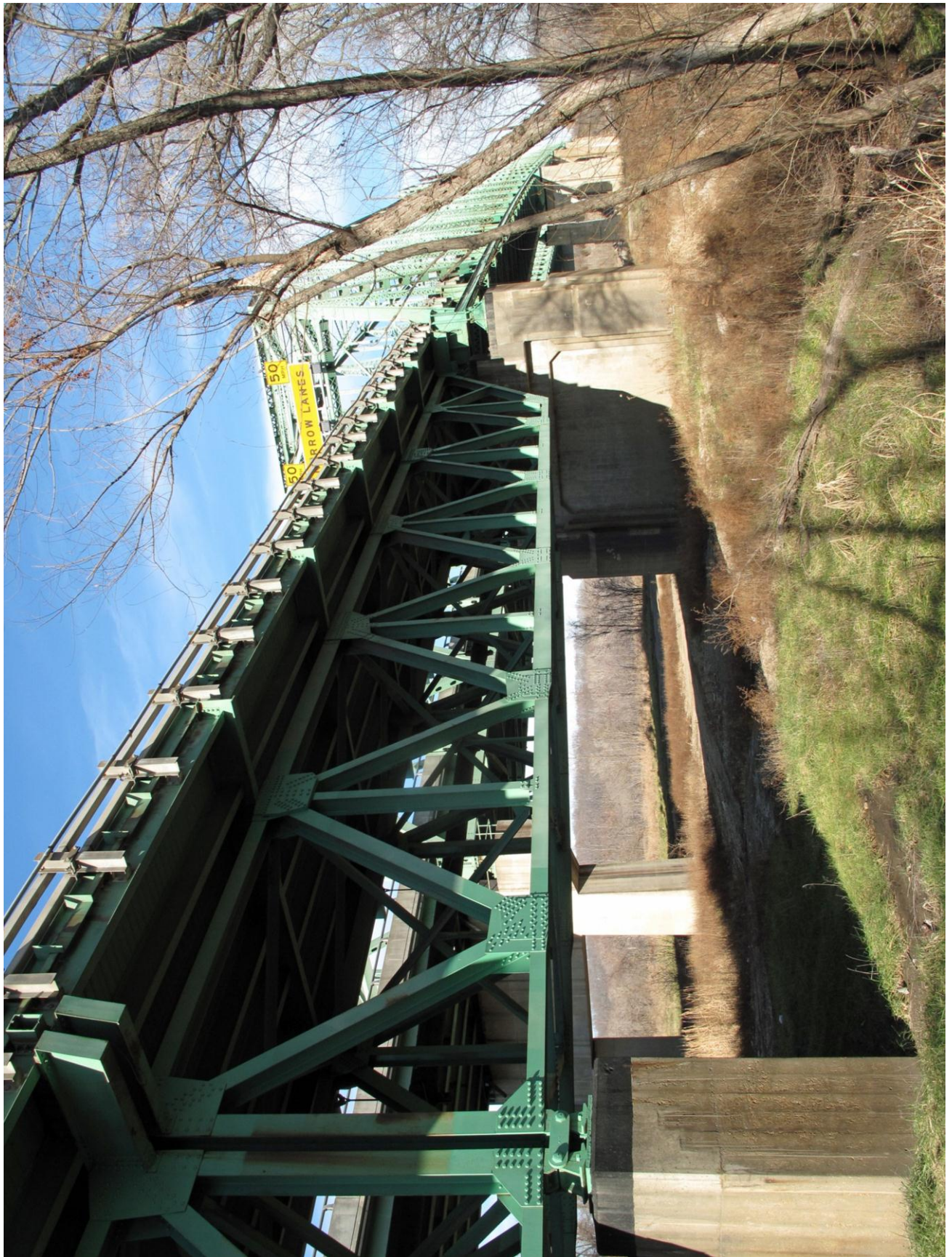
#11 of 27: Facing northwest, span 7 deck truss approach span.
