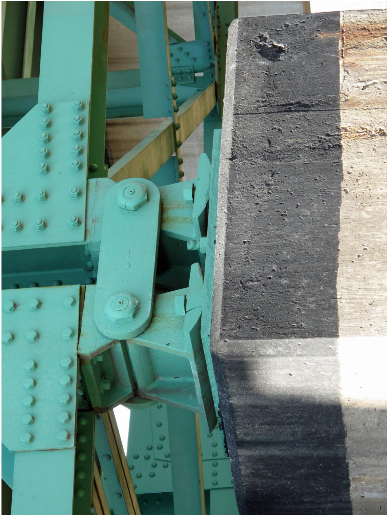
#25 of 27: Facing southwest, rocker bearings on pier 8.
