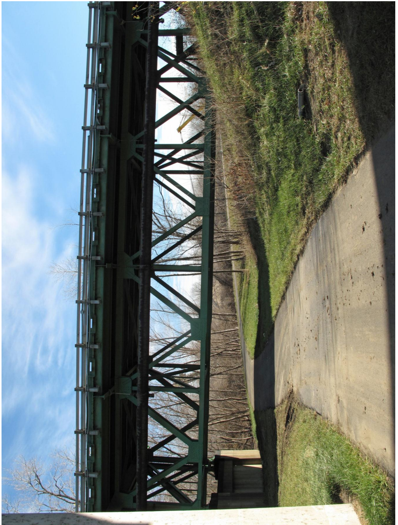
#13 of 27: Facing east, span 8 deck truss approach span.
