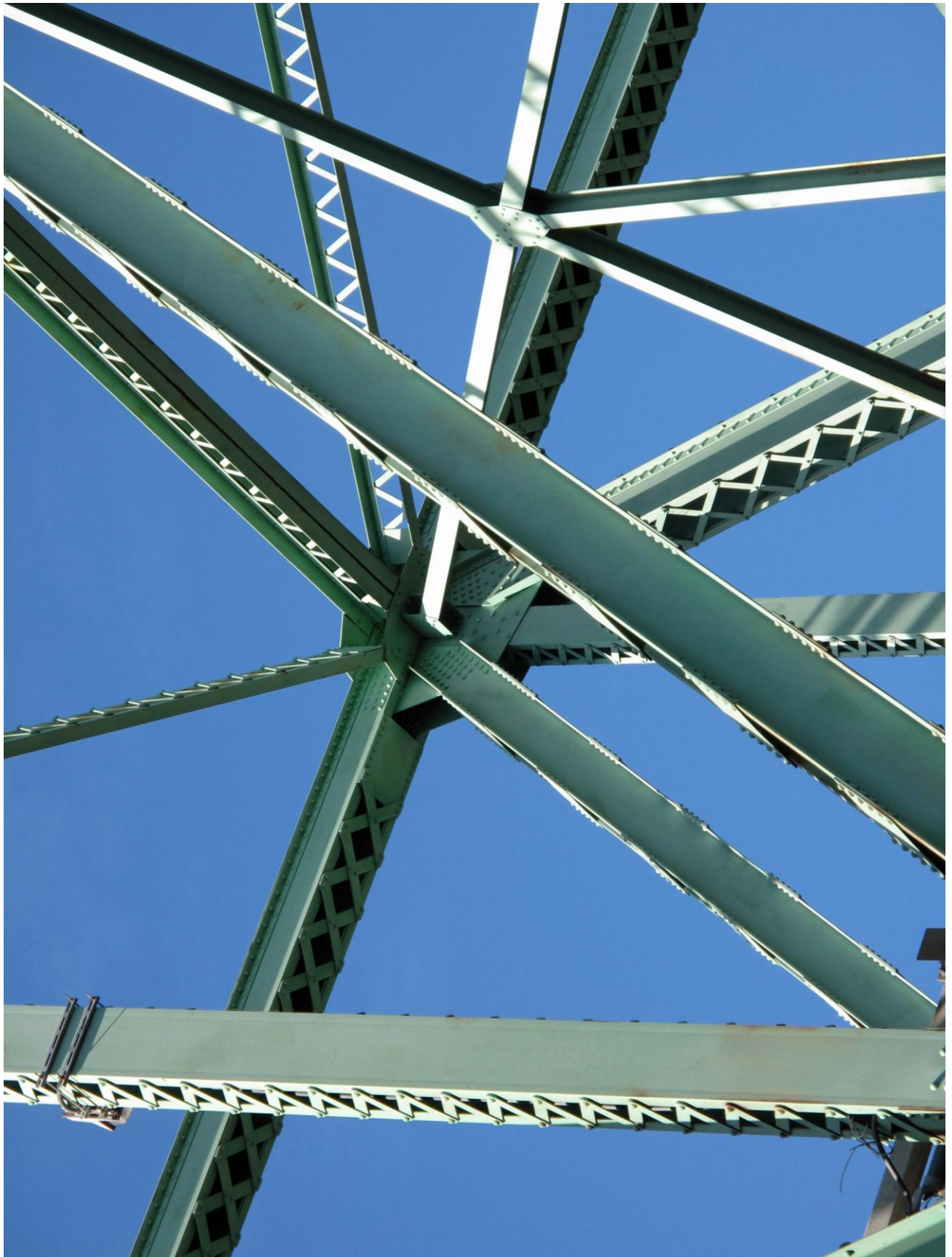
#24 of 27: Facing west, detail of connection between side panel, top chord, lateral bracing and sway bracing.
