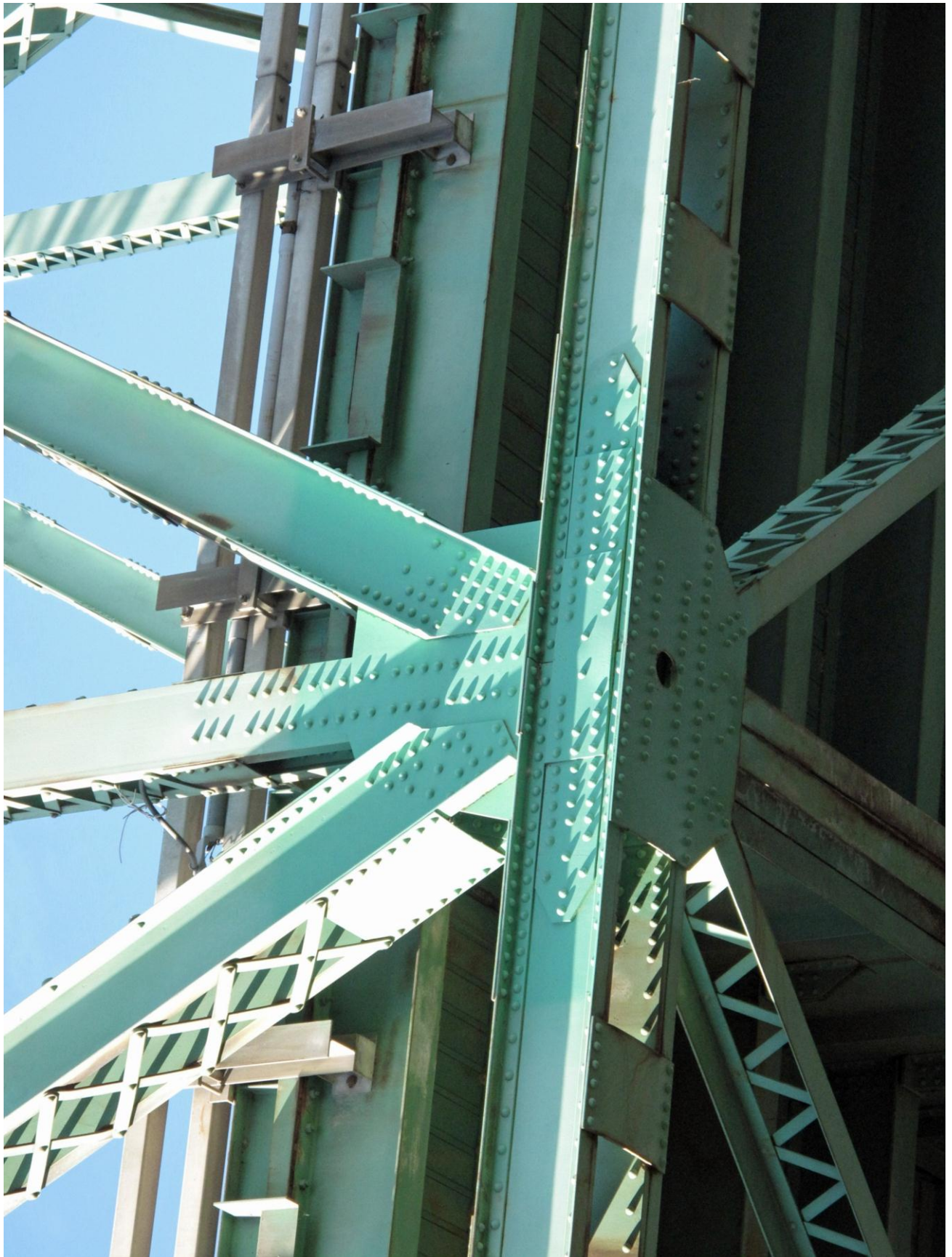
#23 of 27: Facing west, detail of connection between side panel and bottom chord.
