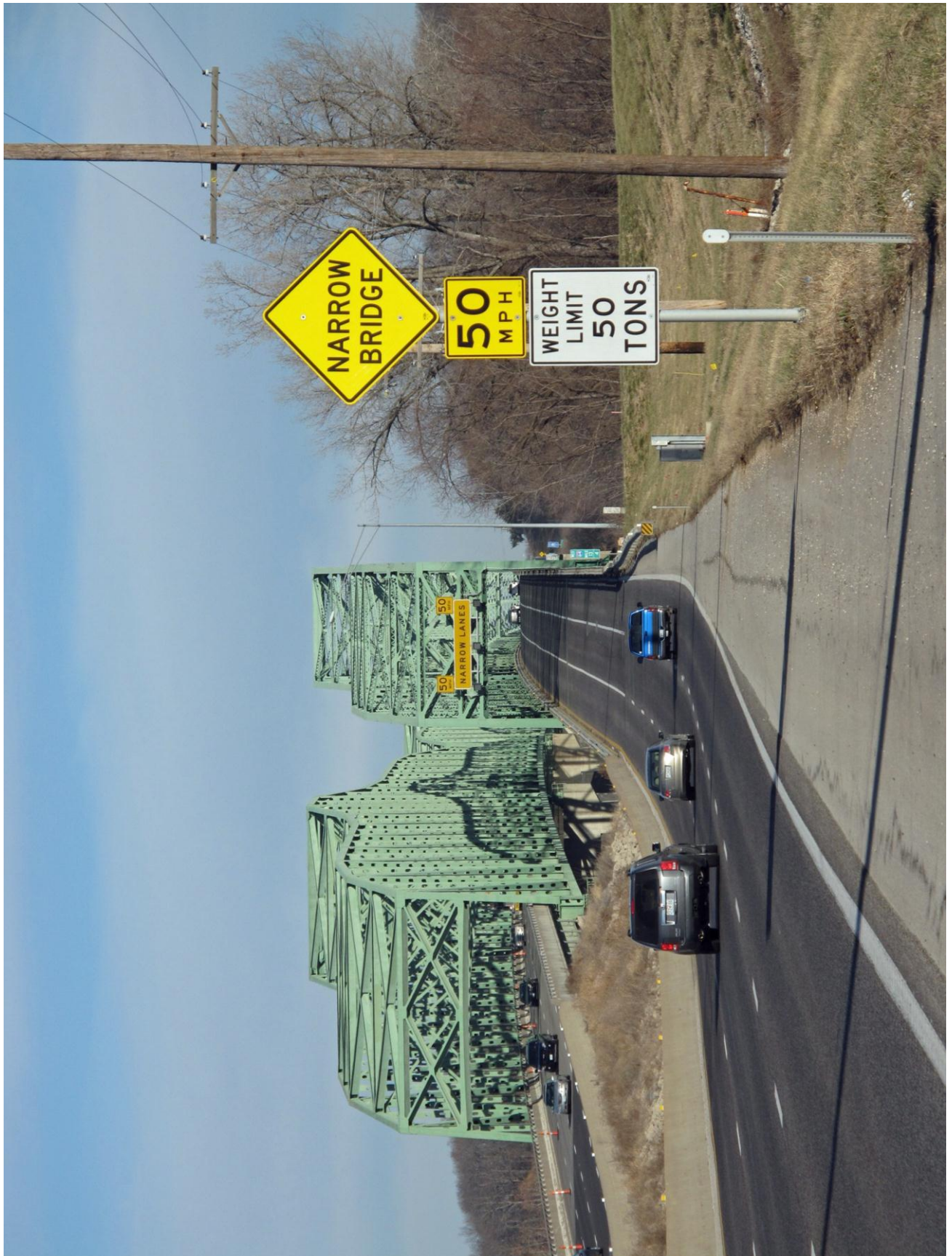
#8 of 27: Facing north, South portal of through truss span; includes companion bridge A4017; notice the shadow cast by the polygonal top chord onto the companion bridge.
