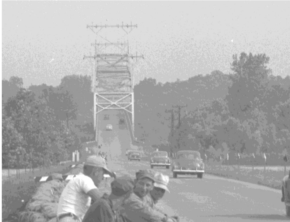
Figure 12: Daniel Boone Bridge, showing original configuration of portal bracing.
