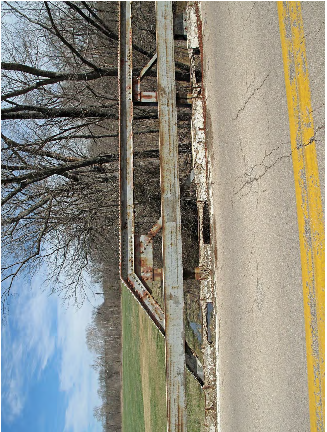
5 of 24. St. John's Creek Bridge, N0141, facing northeast, span 1, Pratt pony truss, panels 1-3
