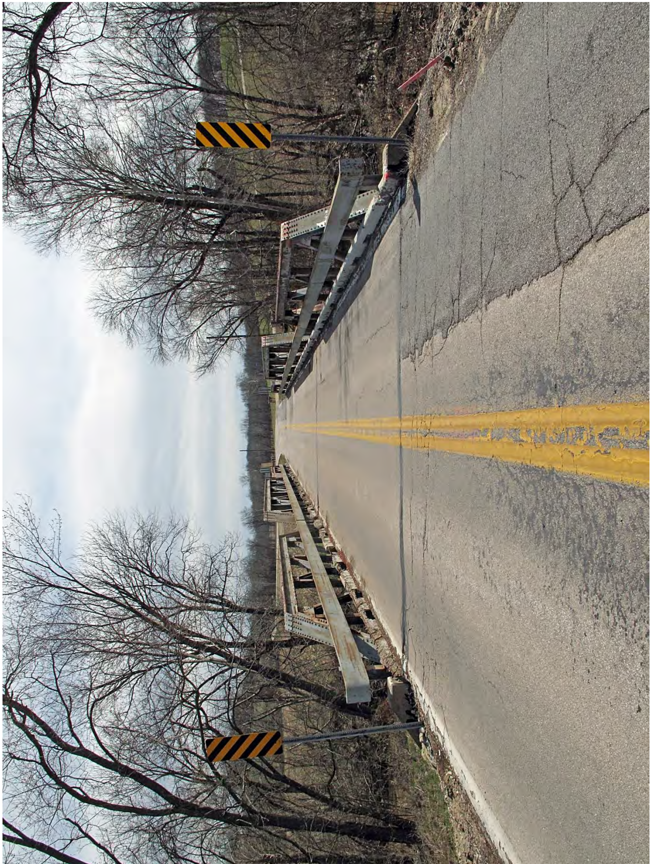
2 of 24. St. John's Creek Bridge, N0141, facing southeast, pony truss spans
