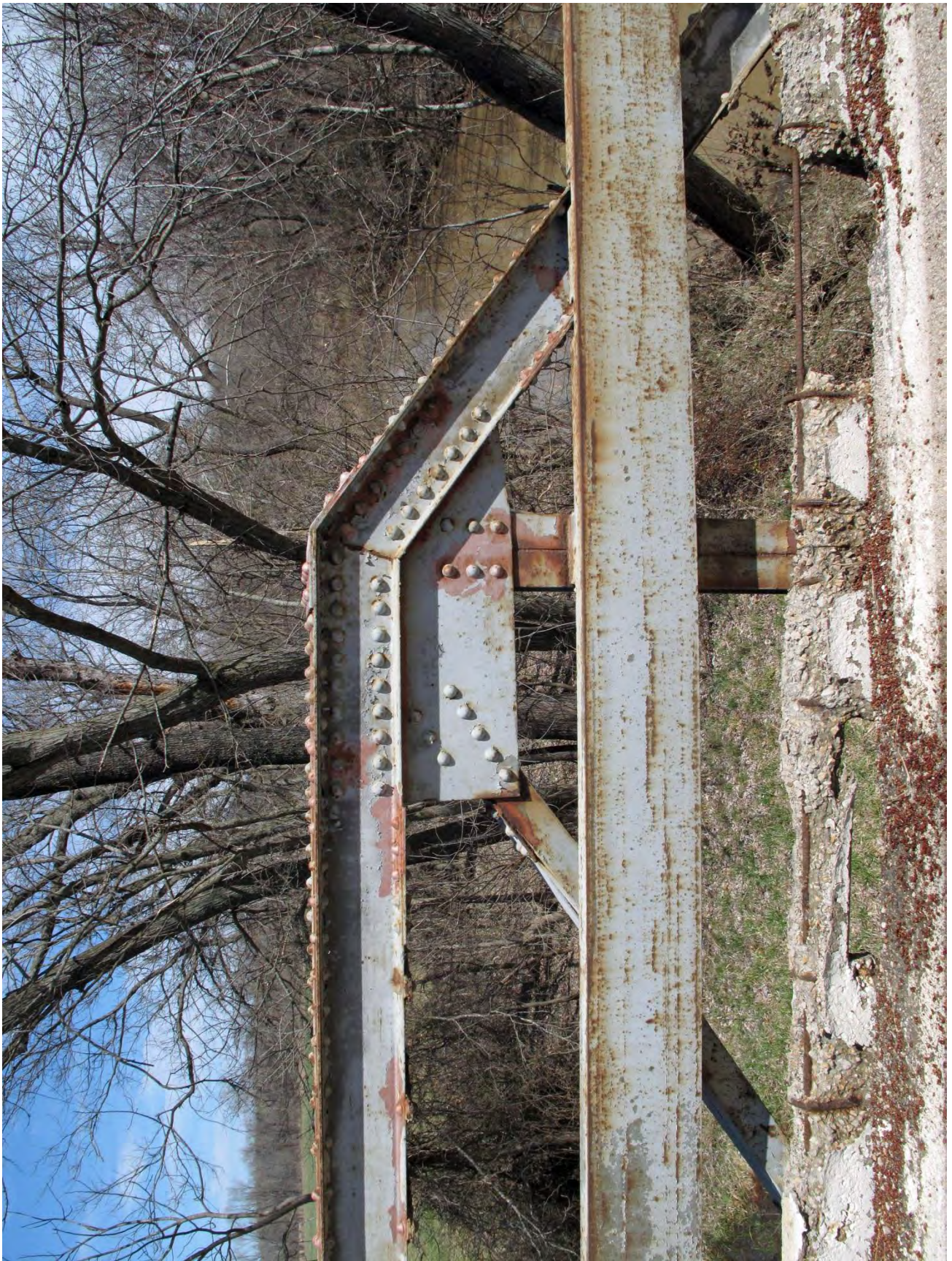
8 of 24. St. John's Creek Bridge, N0141, facing northeast, span 1, detail, gusset plate, inclined end post
