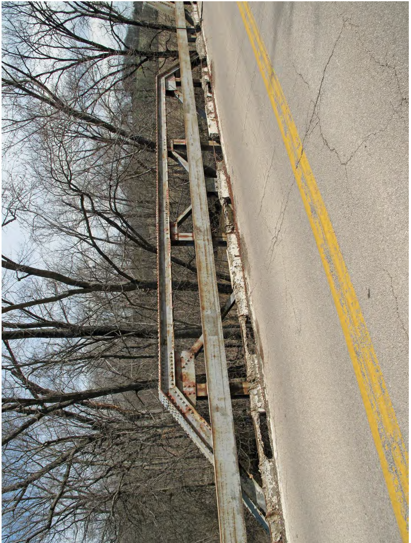
4 of 24. St. John's Creek Bridge, N0141, facing northeast, span 1, Pratt pony truss, northwest end of bridge, northeast truss
