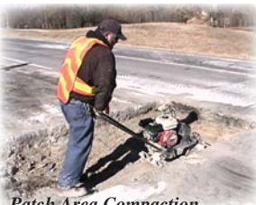
Patch Area Compaction
