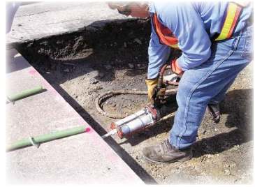
Injecting Epoxy
